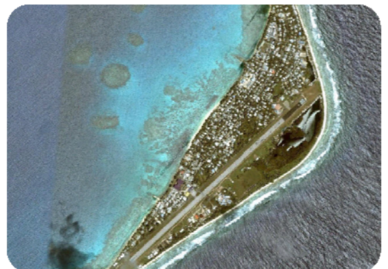
Densely populated Funafuti where solar street lights will be installed
