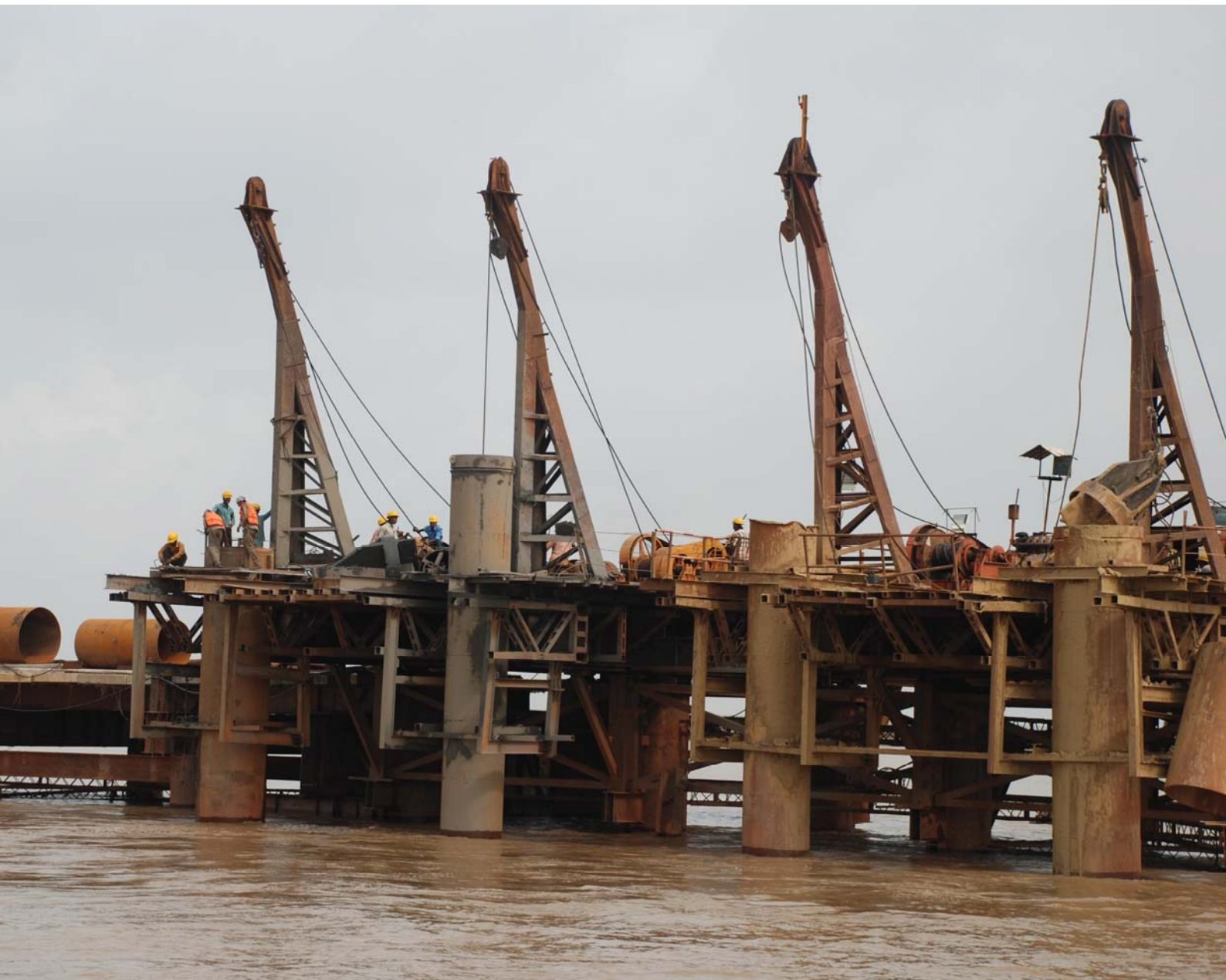
Construction work in progress at Dhamra © IUCN
