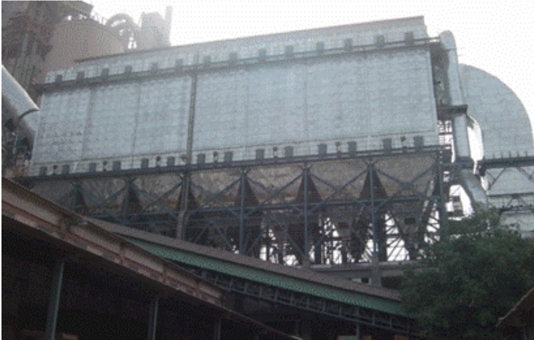
Bag Houses: Reducing & Re-using ©ACC Ltd
