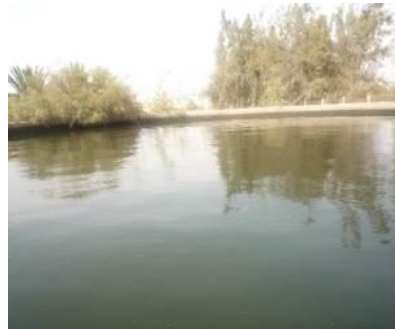
Storage basin CRDA, 1000m3 Water distributor
