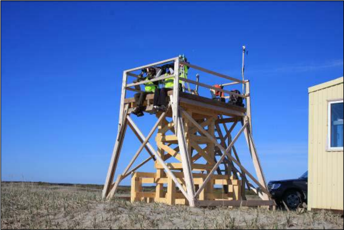
Figure 2. Shore-based behavioral observation team tower. Note second tower within first, designed to balance and steady theodolite readings.
